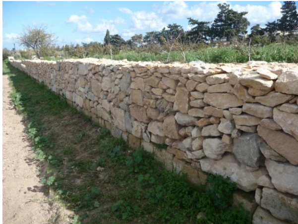
Photo 3. Typical Mediterranean stone retaining wall in Malta. (A protected landscape characteristic).
