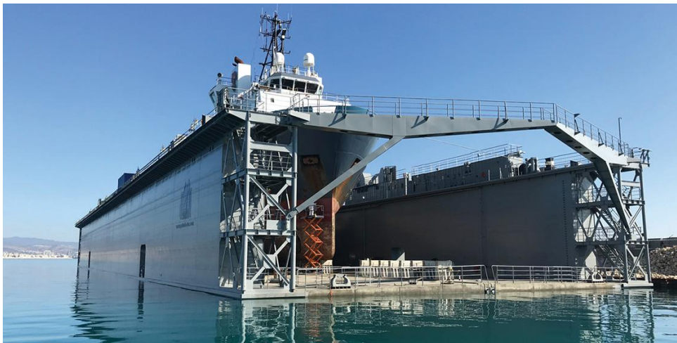
Figure 1 Floating Dock ERENEOS Installed at the Limassol Port
