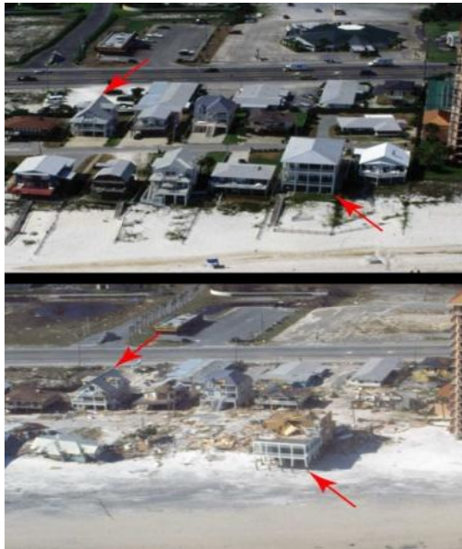
Picture 3. Results of a storm surge produced by Hurricane Katrina's strike - Orange Beach, Alabama. Image by USGS (the arrows show the specific buildings before and after the storm).
